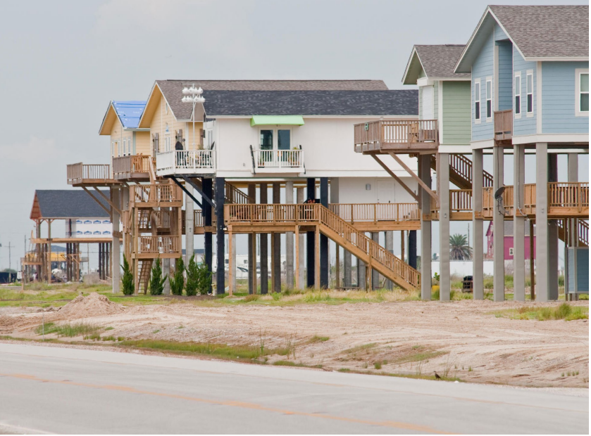
Homes that survived the ~20-foot-high storm surge of Hurricane Ike in Bolivar Peninsula, near the community of Caplen. Image: TWDB
